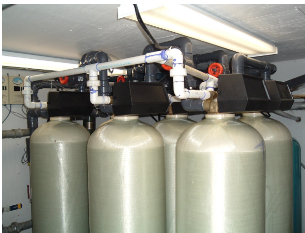
60 GPM Sch 40 Wellwater Configuration at Wagners Greenhouses, Mpls., MN.
