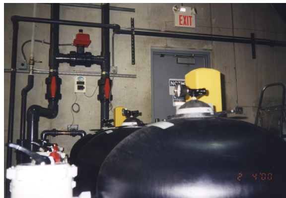
Headered Glass Pack® filters allow reuse of the wastewater, 90 GPM.
